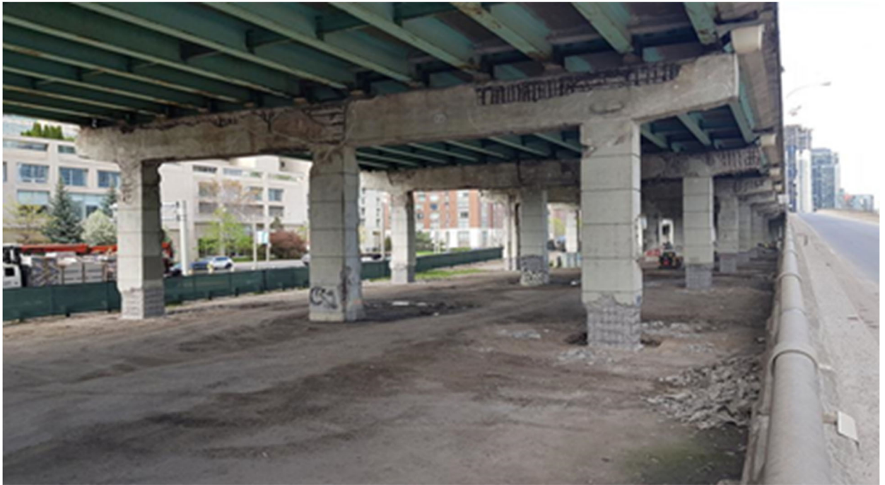
Figure 2: Pier Corrosion Due to Chloride from Leaking Joints and Roadside Splash
