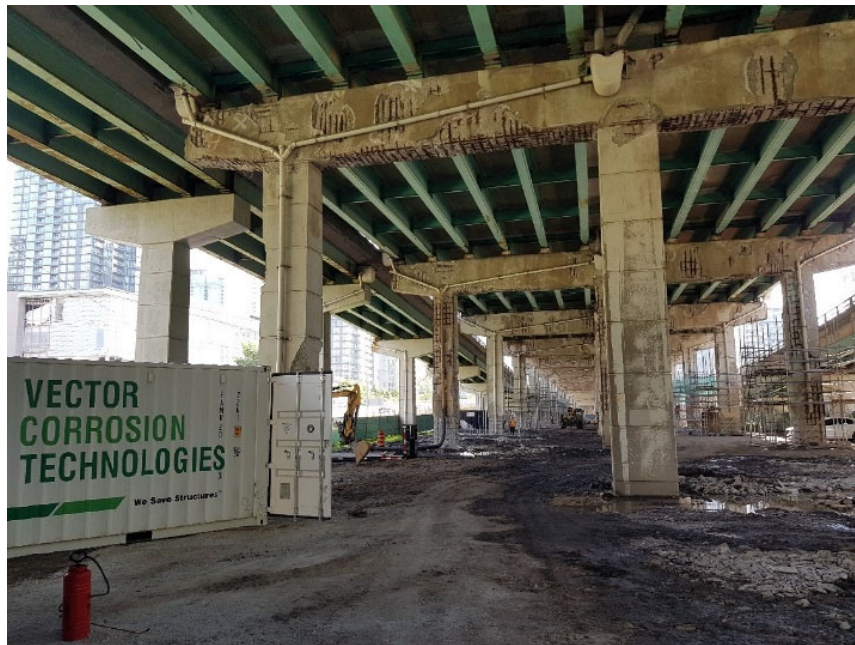
Figure 5: Corrosion Damage of Columns and Pier Caps with Patch-Accelerated Corrosion Evident
