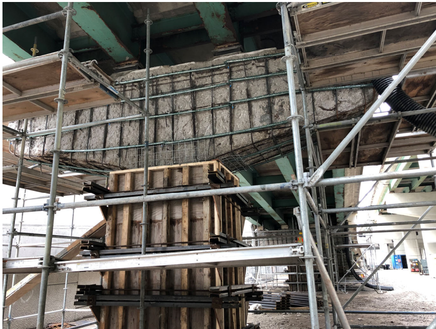
Figure 9: Galvanic Encasement for Hammer Head Pier (Green “bars” are the Distributed Galvanic Anodes)
