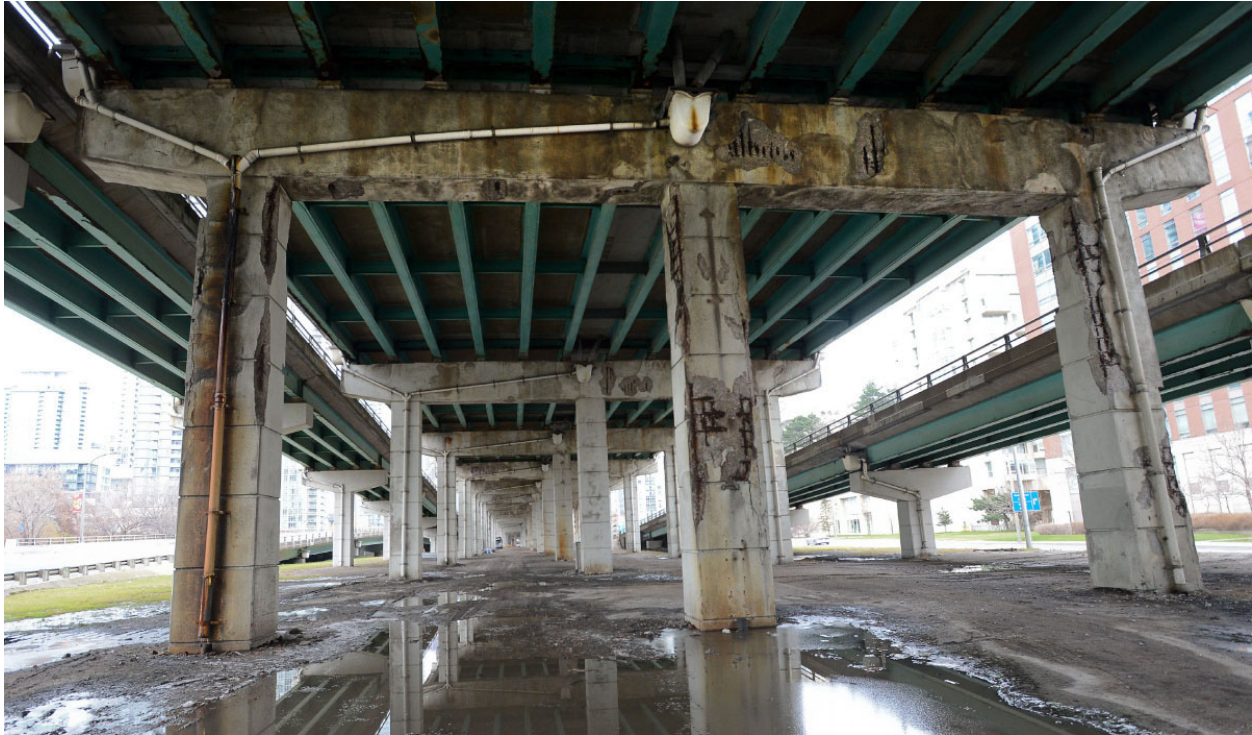
Figure 1: Pier Concrete Corrosion due to Leaking Expansion Joints and Chloride Contamination
