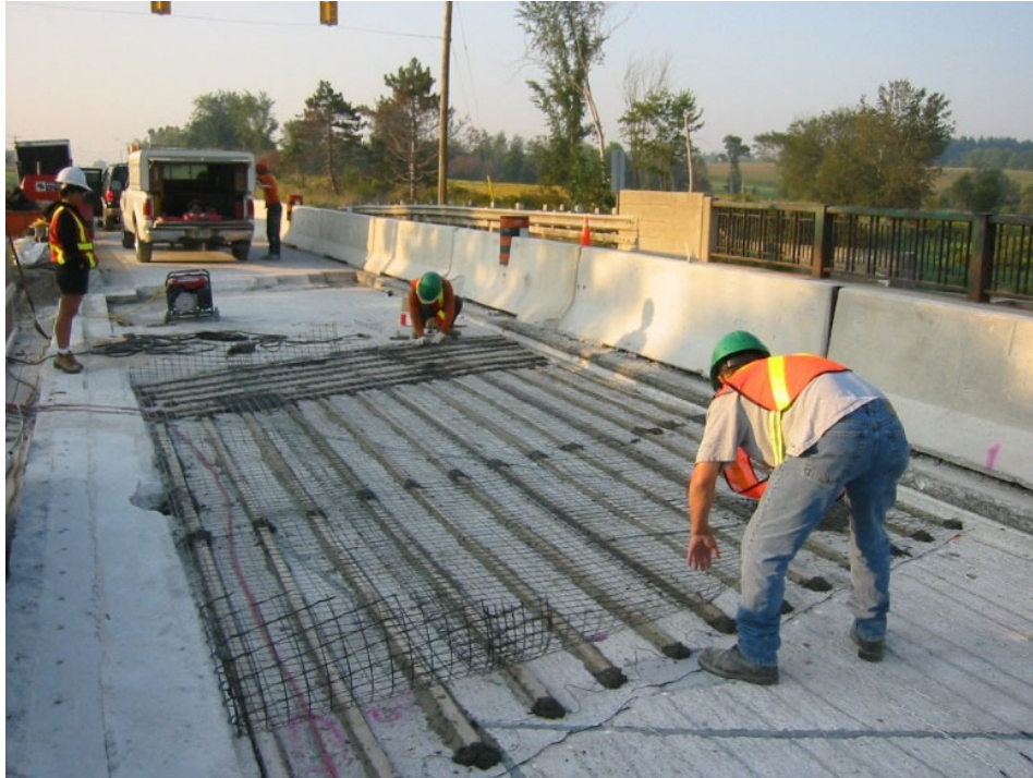
Figure 3: First installation of distributed galvanic anodes on a bridge deck prior to bridge deck overlay, Ontario, Canada, 2003
