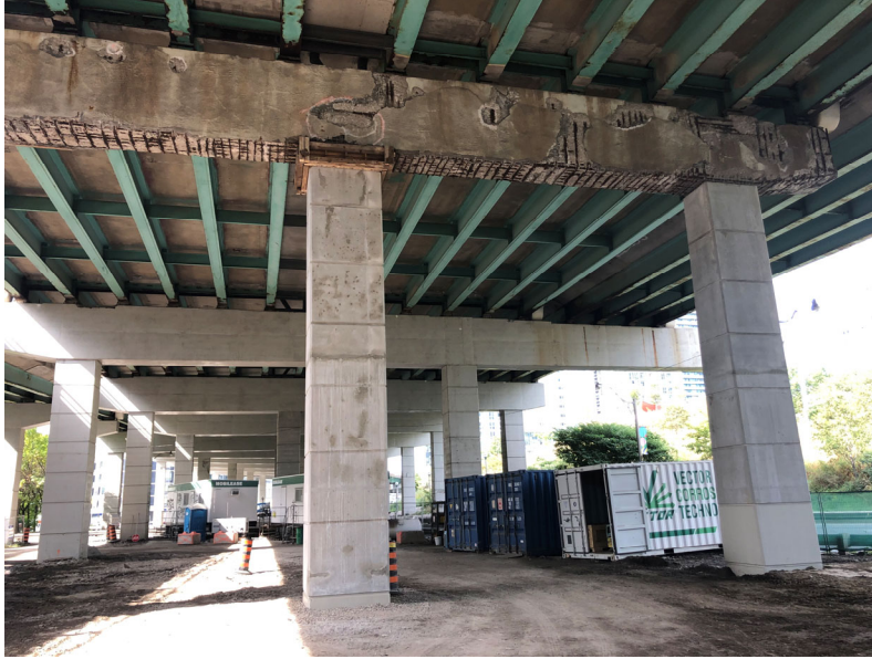
Figure 10: Completed Piers in the Background with a Partially Completed Pier in the Foreground
