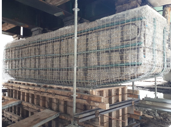
Figure 8: Galvanic Encasement Details
