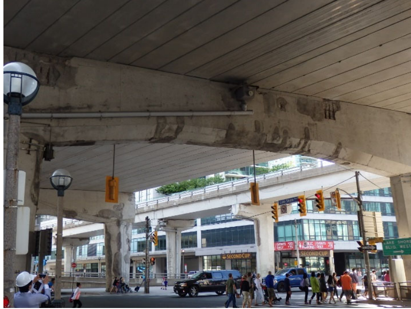
Figure 4: Corrosion Damage of Columns and Pier Caps with Patch-Accelerated Corrosion Evident
